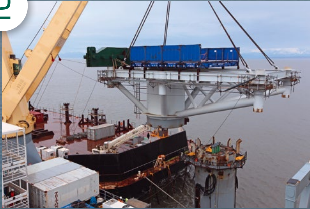
Installation of transition piece
