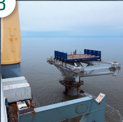
Transition piece installed
