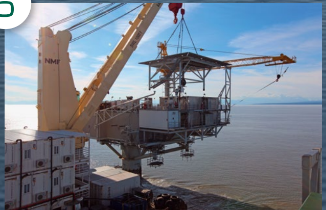
Installation of helideck
