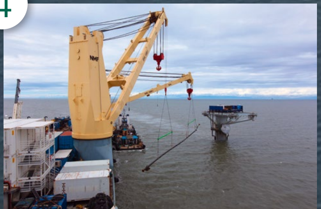
Finishing of pipeline connection
