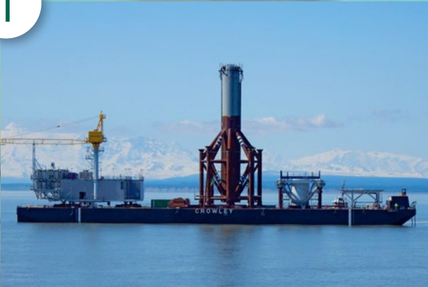
Barge arrives with monopod, transition piece, topside and helideck
